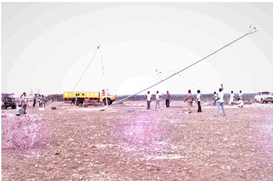
Figure 4. Installation of the first mast under National Wind Monitoring program in 1984
