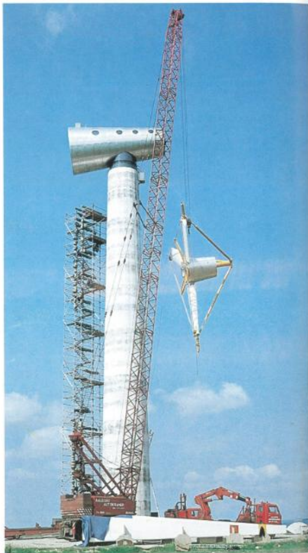
Mounting of the rotor on the Nibe A turbine. 1979.
