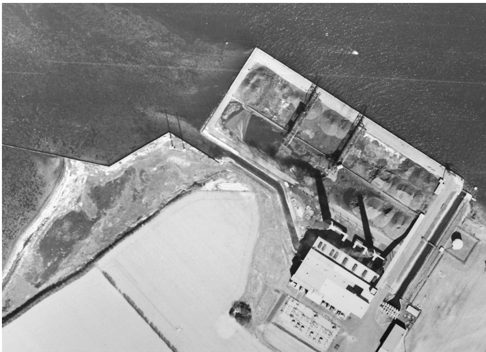
Figure 5: Same as above, only zoomed onto the power plant. The power line lattice tower that was (likely) used for this experiment, is visible to the North-West of the plant. See also Figure 6. Source: https://map.krak.dk .
